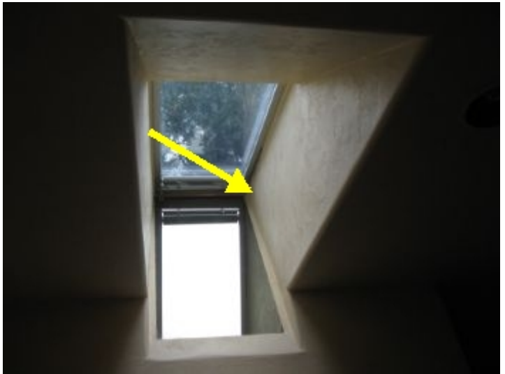
Skylights in home (4) are all installed correctly as seen and flashed properly. No evidence of any leakage at the time of inspection.
