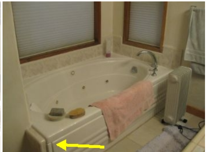
Whirlpool tub in master bath properly wired with GFCI breaker and access to pump and heater systems from front Tile around in great condition as well as woodwork which is water protected and walls.
